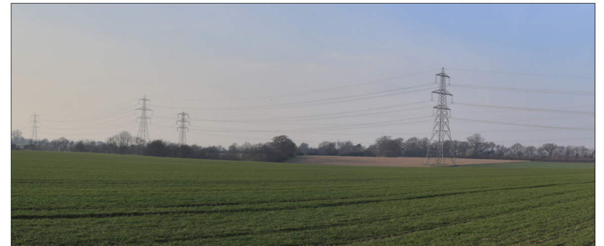
Alternate view of overhead lines to the north, approximately 500m west of the viewpoint.
